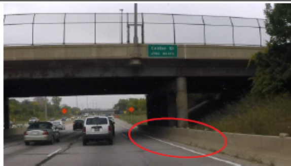
Southbound IH 43 - Center Street Bridge -Less than 10-foot paved shoulder under structure -Beam guard and concrete barrier
