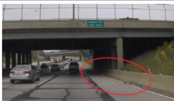
Southbound IH 43 - Capitol Drive Bridge -Less than 10-foot paved shoulder under structure
