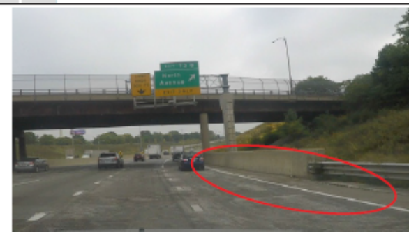
Northbound IH 43 - Brown Street Bridge -Approximately 10-foot paved shoulder with face of curb barrier wall and inlets
