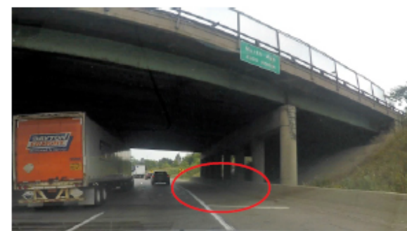
Northbound IH 43 - North Avenue Bridge -Less than 10-foot shoulder under structure
