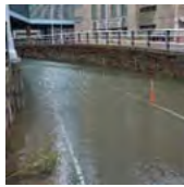
Hurricane Sandy Project
