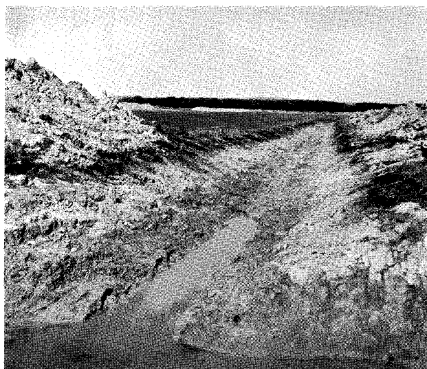
Surface drainage, properly designed, will lower water tables and permit the use of wet soils for cultivated crops.
