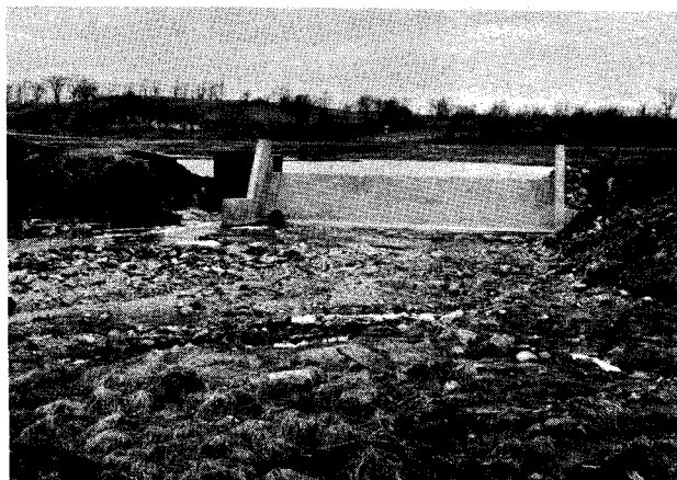
An embankment that failed because of soil piping.
