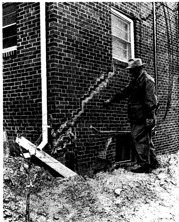
Poor shear strength and bearing capacity and high shrink-swell potential in soils can crumble foundations and topple buildings.
