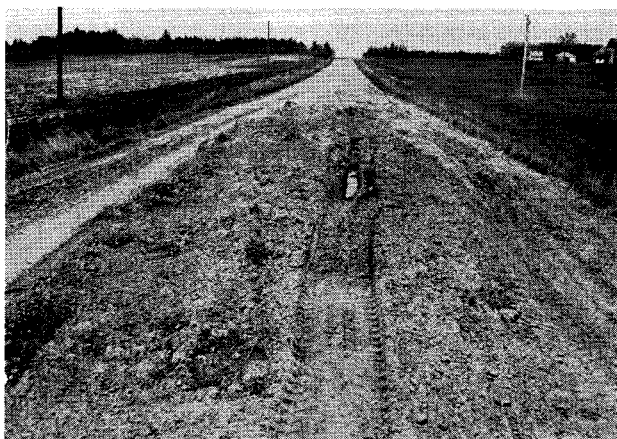
Frost heaving is a real hazard in silty, somewhat poorly drained soils. Frost boils turn to mud holes such as this.
