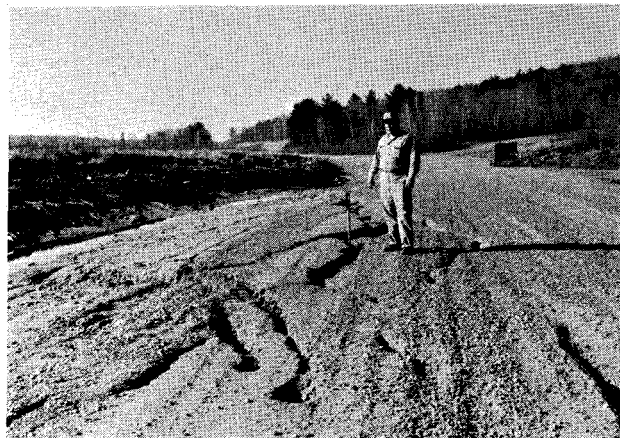
The base for this failing roadway is organic materials such as those that comprise the Houghton mucky peat soil profile.
