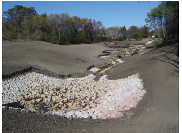
Photo 19 Stream rehabilitation in progress along a formerly concrete-lined channel.
