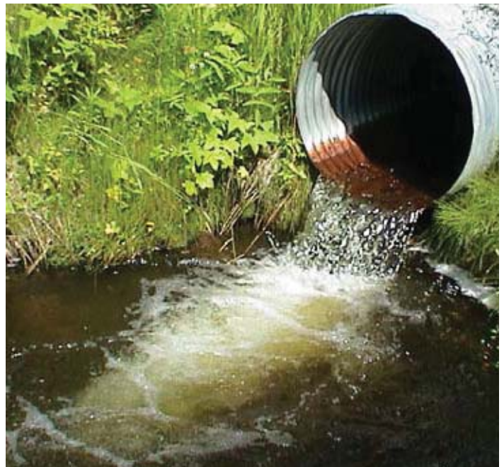
Photo 17 Perched culvert outlet blocking passage of aquatic organisms from downstream to upstream.
