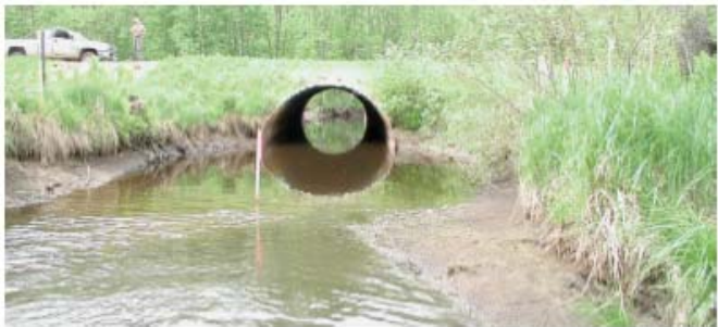
Undersized culvert.
