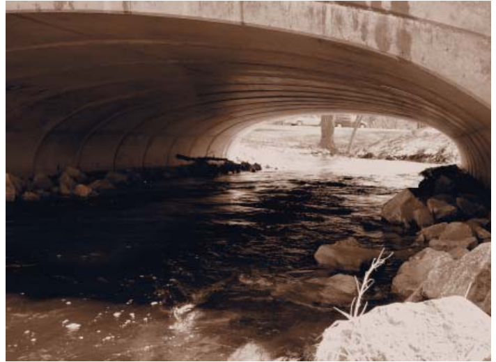
Photo 16 Bridge crossing with naturalized bed enabling passage of aquatic organisms.
