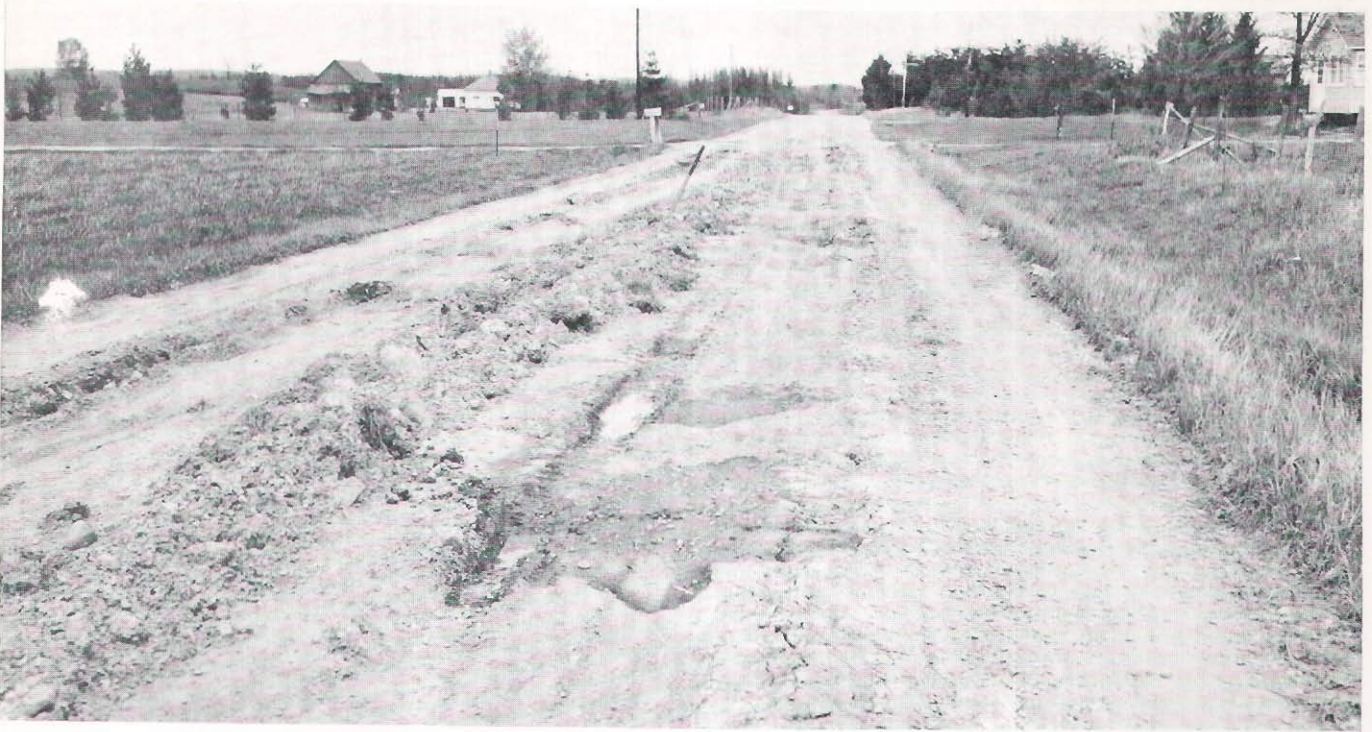
Figure 21 FROST HAZARD ACTION
