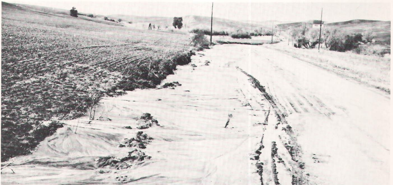
Figure 17 SILTING OF DRAINAGE DITCHES
