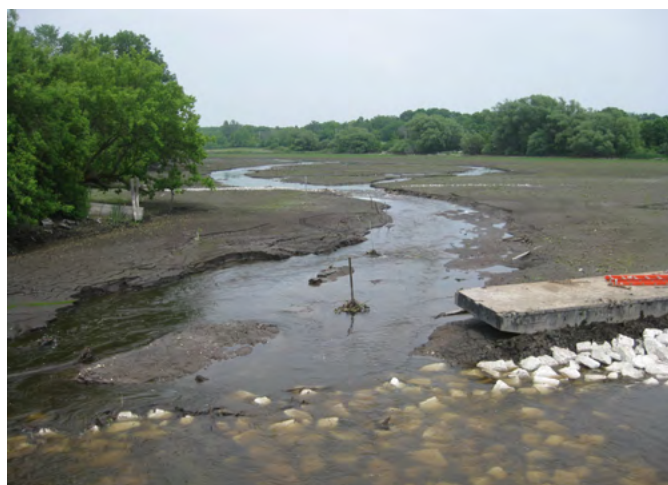
Figure 2.16 Monches Dam Millpond During Drawdown Condition: June 2013
