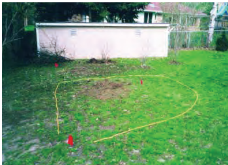
The perimeter of a rain garden is defined with string before digging.
