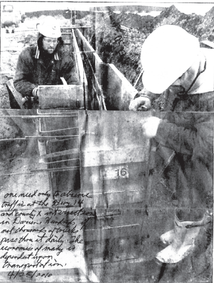
Brian Reynolds, left, and Aaron Zimmerman set forms for a section of the foundation of the Professional Power Products building being erected in Darien's industrial park.
