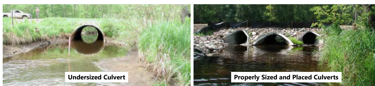
Figure E.2 Considerations for Culvert Design and Placement
