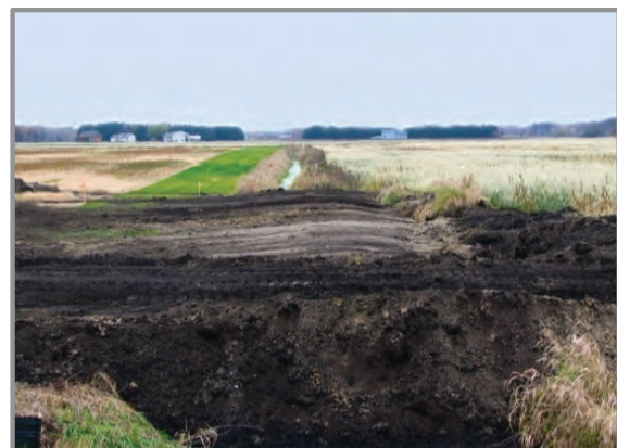
Figure 12. Finished Ditch Plug with Crown in Middle
