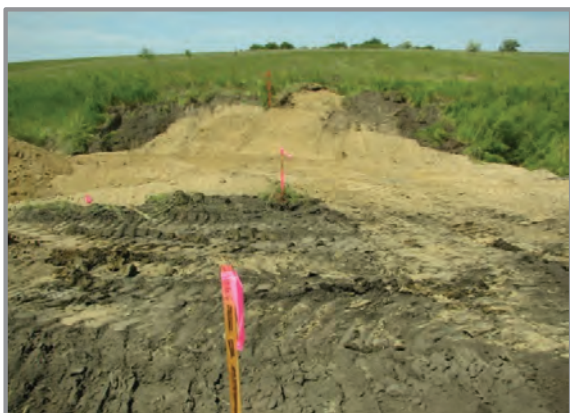
Figure 10. Ditch Plug under Construction
