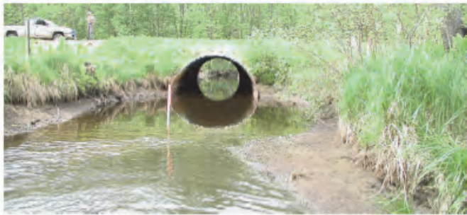
Undersized culvert.
