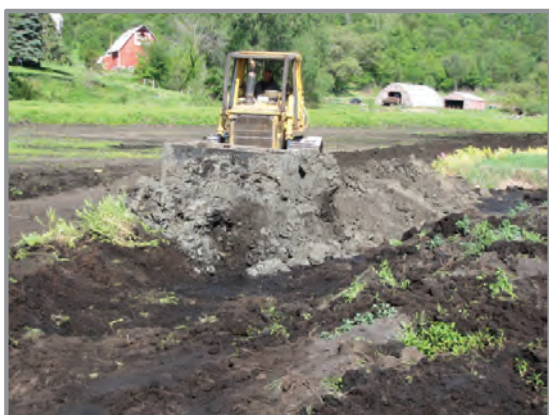
Figure 2. Shallow Ditch Being Filled
