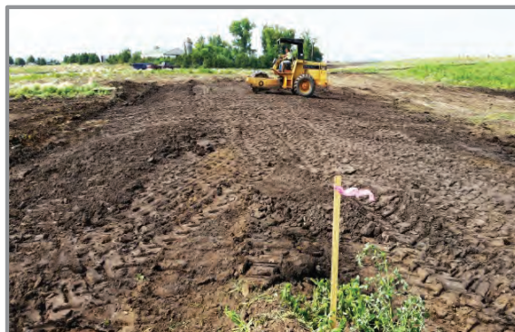
Figure 11. Compaction of Constructed Ditch Plug
