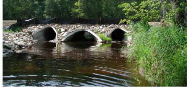
Properly sized and placed culverts.
