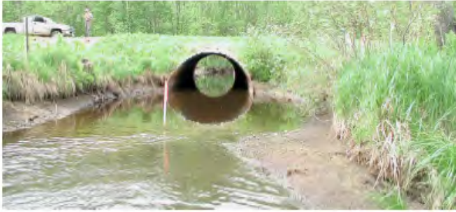
Undersized culvert.
