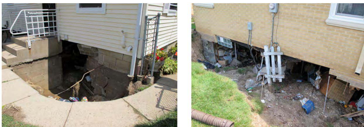
Figure 3.6 Damage to Residential Property Caused by the July 2010 Flooding
