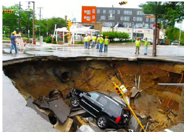
Figure 3.5 Sinkhole Resulting from Flooding near North Avenue and Oakland Avenue, July 21, 2010
