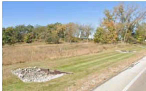
Figure 3.8 Regenerative Stormwater Conveyance Along Hwy 67
