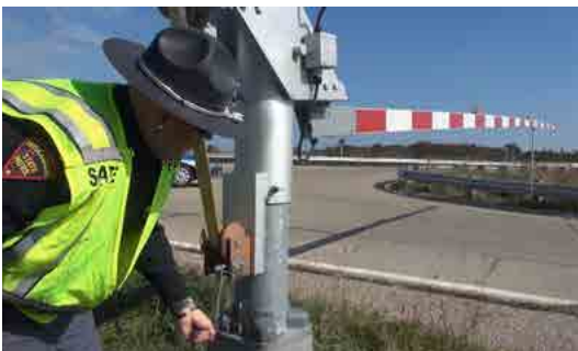
A Ramp Closure Device Credit: WisDOT
