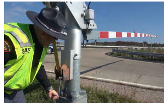
A Ramp Closure Device Credit: WisDOT
