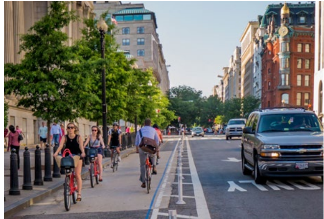
A two-way protected bike lane utilizing bollards in Washington, DC Credit: Stewart Eastep
