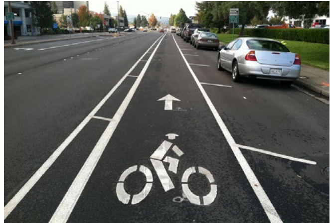
A buffered bike lane that utilizes a buffer zone on both the travel lane and parking lane sides in Kansas City, Kansas Credit: Bike Walk KC
