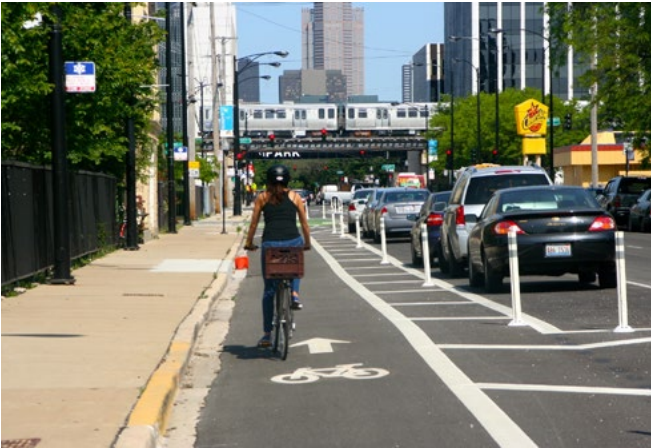
A one-way protected lane utilizing bollards to create separation for bicyclists on Kinzie Street in Chicago, Illinois Credit: Chicago Department of Transportation
