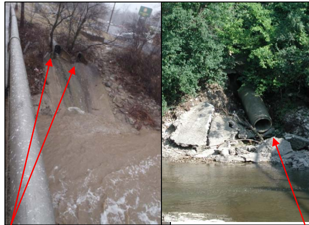
Horlick Dam Northwest (left, both discharge points) and East outfalls (right). East outfall end pipe has disconnected from discharge point.
