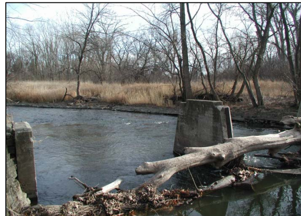
Deteriorated concrete pillars do not appear to be functional , are collecting large debris and should be investigated for removal.
