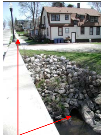
Uphill sanitary sewage source (left arrow) and southeast outfall (right arrow).
