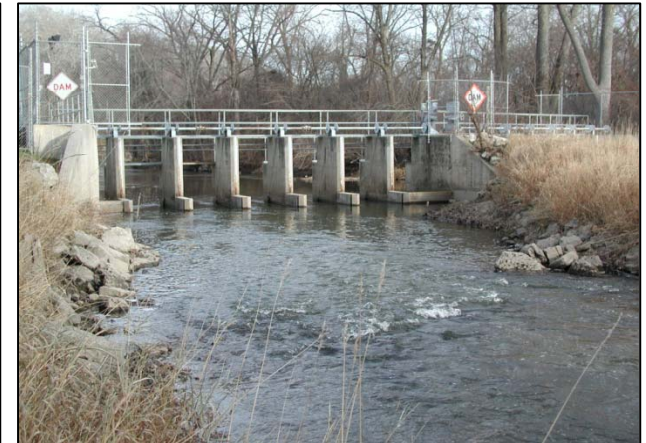
Looking downstream from sampling location in winter. Fish weir runs across stream width and free-standing rocks stabilize nearby banks.
