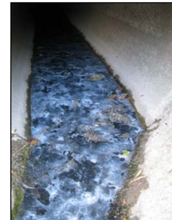
High levels of detergents found in southeast outfall (note foaming present in storm water discharge).
