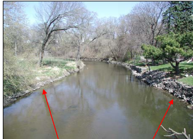
Looking upstream from sampling point in spring. Moderate rock support on west (left) bank and established rock walls on east (right) bank.
