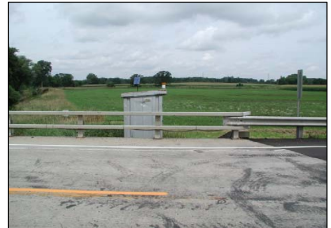
U.S. Geological Survey Discharge Gauging Station on east (right) bank provides continuous volumetric flow rate measurements.
