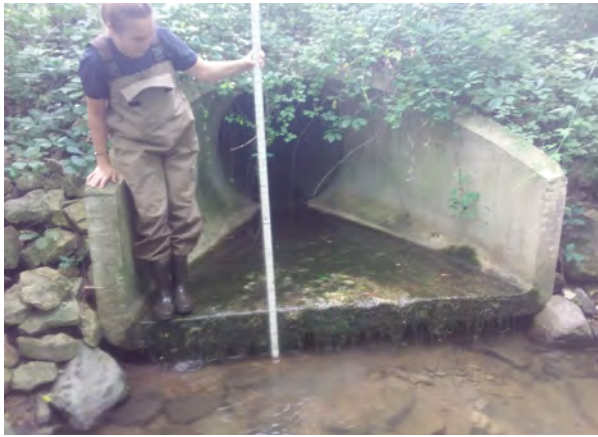
Figure 4.71 Algal and Plant Growth on Stormwater Outfall Discharging into Oak Creek near W. Thorncrest Drive: July 25, 2017
