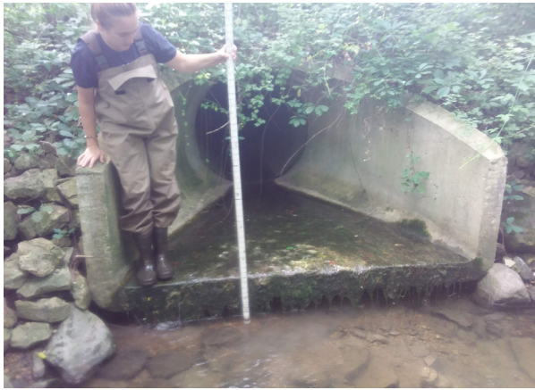
Figure 4.X Dissolved Oxygen-5 Algal and Plant Growth on Stormwater Outfall Discharging into Oak Creek near W. Thorncrest Drive: July 25, 2017
