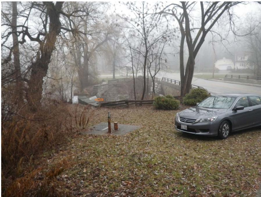
Photo 6: Dam Spillway at arrow. Crank for low level gate operation in concrete pad, foreground.
