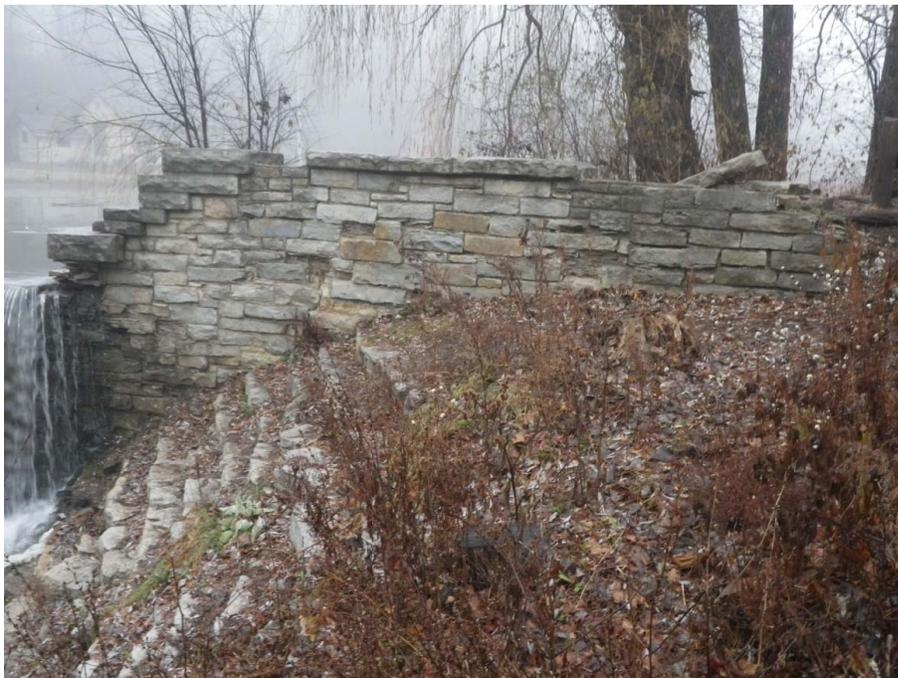
Photo 14: Left abutment downstream face and stone paving on downstream slope
