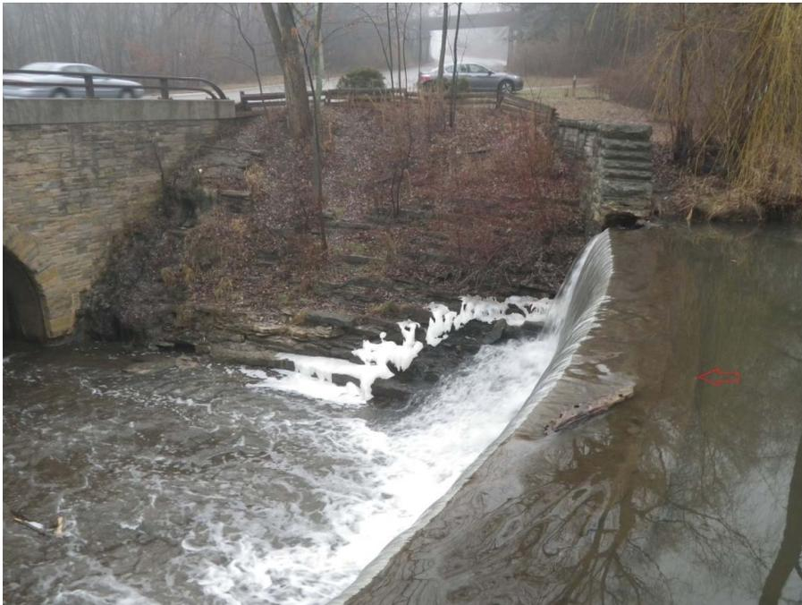
Photo 4: Right Embankment between Spillway and Mill Road Bridge. Note concrete wall at curved spillway, arrow.
