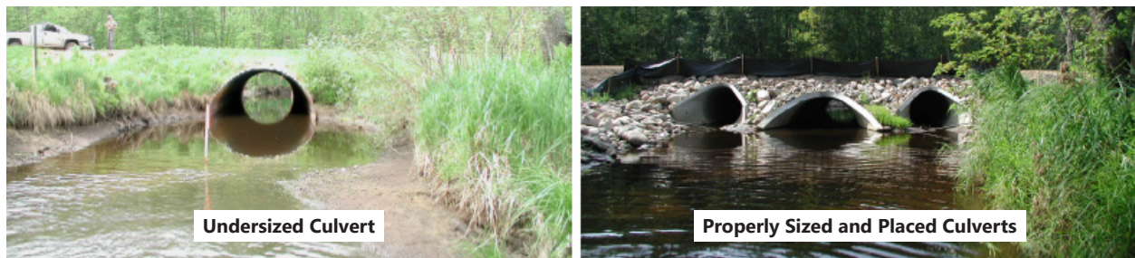
Figure Y.1 Considerations for Culvert Design and Placement
