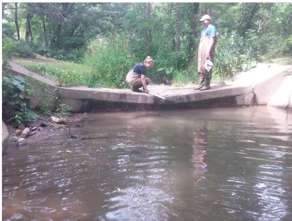
Structure Number 52 Concrete Weir Crossing Oak Creek
