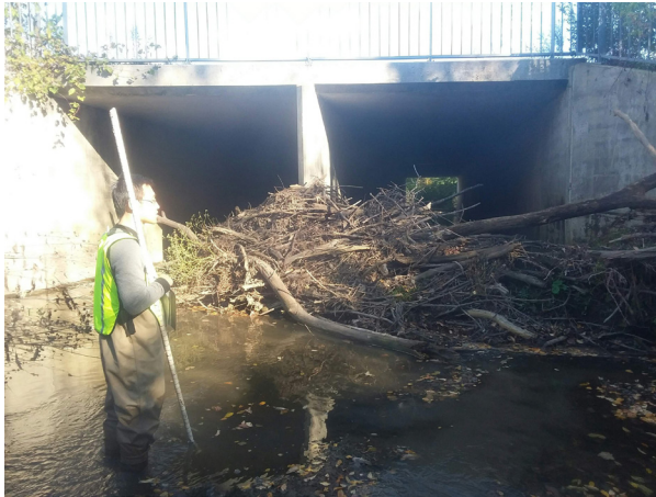
Figure 4.30 Large Debris Accumulations on Oak Creek at the Shepherd Avenue Culvert: 2016
