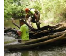
Selectively Remove Parts of Woody Debris to Open Passage Lanes
