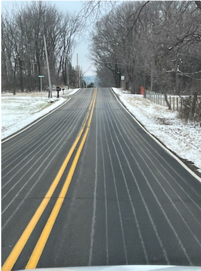
Figure 8.10 Anti-Icing Brine Applied in a Wet/Dry Striped Pattern
