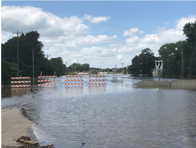
Floodwaters submerging the Highway 50 bridge over the Fox River in the Town of Wheatland
