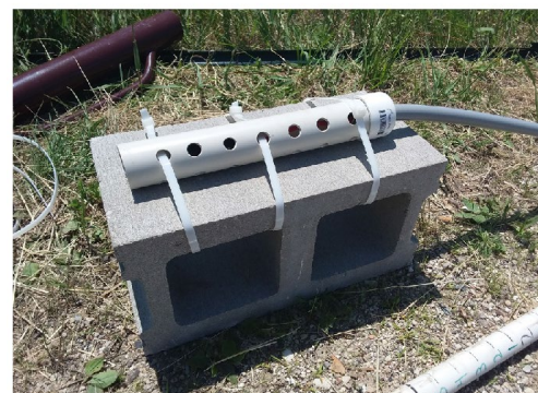
Figure 7.1 Continuous Sensor and Housing Assembly
