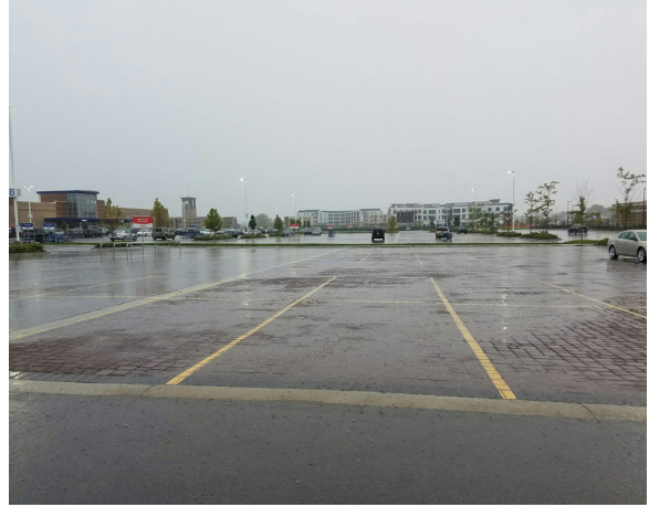
Porous Pavement Infiltrating Runoff from Parking Lot at Drexel Town Square
