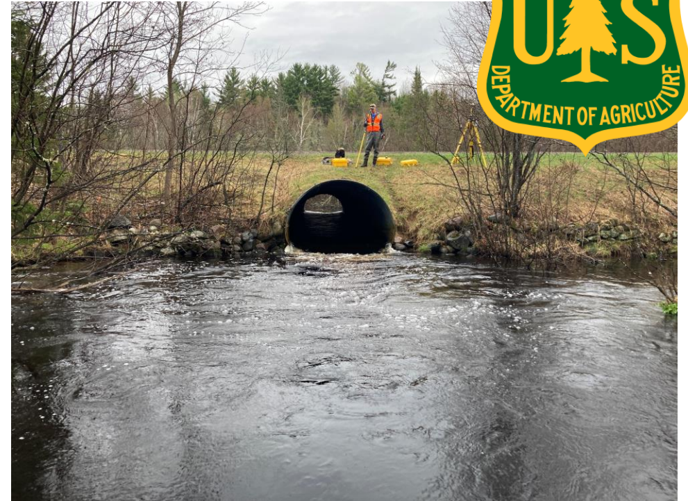
Undersized culvert at Elvoy Creek in Forest County that will be replaced with a 30-ft-wide bridge to restore flows and allow fish passage
