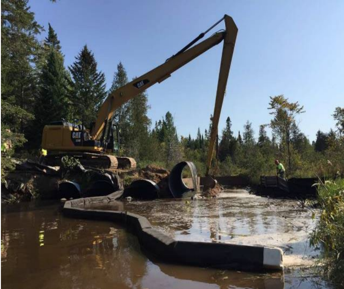
Removing an Aquatic Organism Passage Barrier – Trout Unlimited
