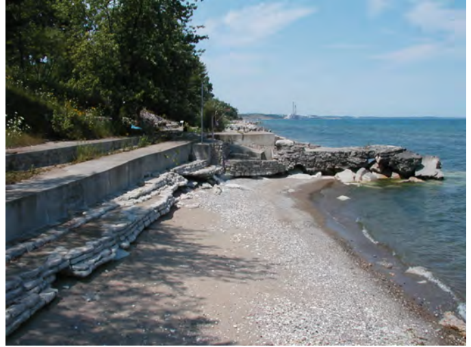
Seawall (in foreground)
