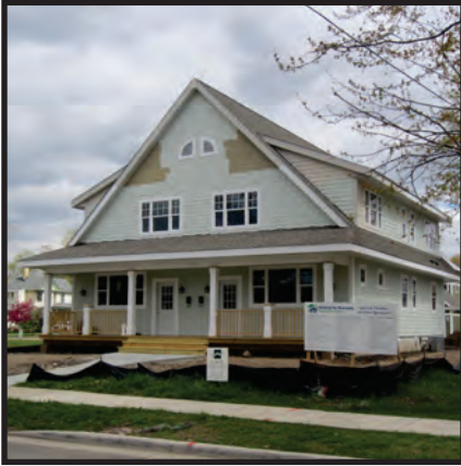
Duplex constructed by Habitat for Humanity nearing completion in the City of Waukesha.
