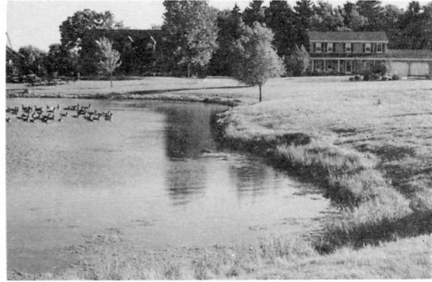
Figure III-20. Stormwater management basins should be graded with gentle side slopes to blend into the landscape.
