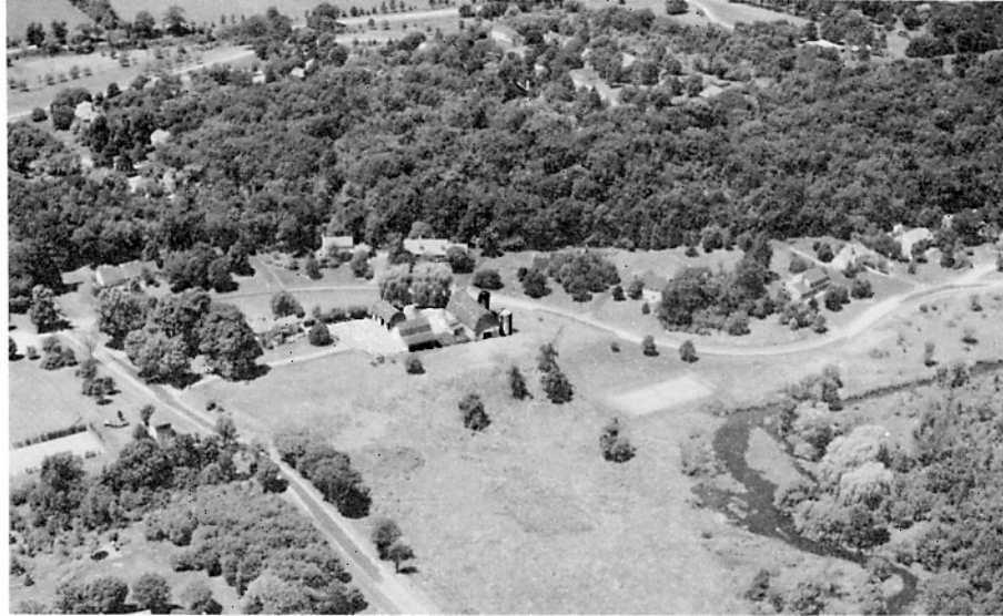
Figure III-24. The barn complex at Woodfield Village in the Town of Merton, Waukesha County, serves as a horse stable and is incorporated into the design as a community asset. It is surrounded by ample open space, preserving rural landscape character next to the perimeter road.
