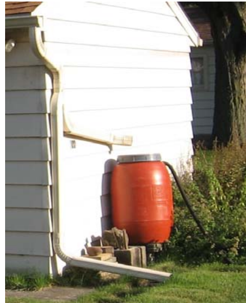
Above: A rain barrel set up to catch rainwater from a gutter. This prevents some rainwater from flooding the streets during a storm.
