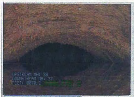
Photo 3-1. Wright Street Storm Sewer, east of Wauwatosa Avenue
