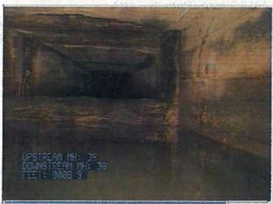
Photo 3-2. Wright Street Storm Sewer (above water)
