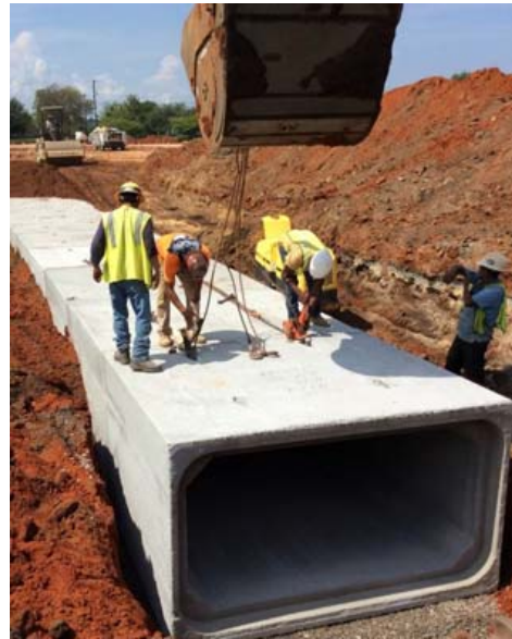
Above: construction workers install a reinforced concrete box culvert, like those used in several of the alternatives. Photo credit: Gossett Concrete Pipe Co., Inc.
