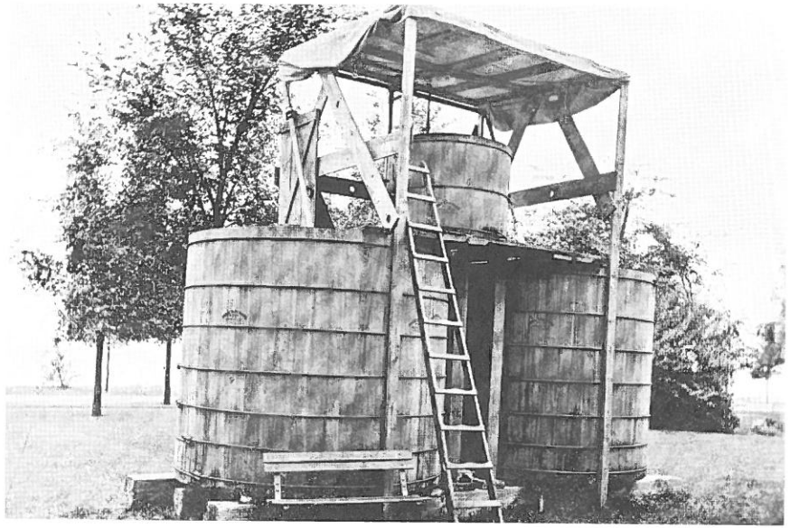
FIRST WATER TREATMENT EQUIPMENT, 1910.
