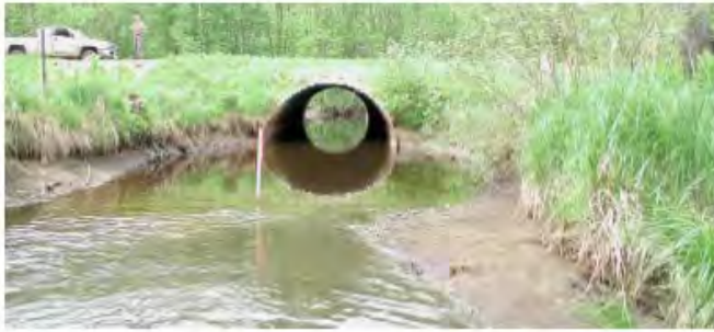
Undersized culvert.
