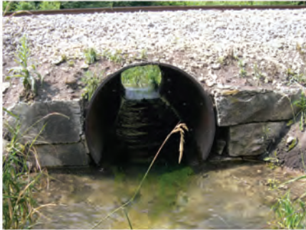
45- WISCONSIN AND SOUTHERN RAILROAD (RM 6.15)
