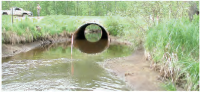
Undersized culvert.
