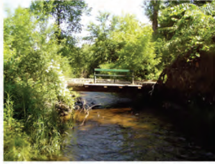
39- FOOT BRIDGE (RM 2.74)
