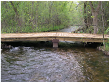
32- FOOT BRIDGE (RM 0.58)
