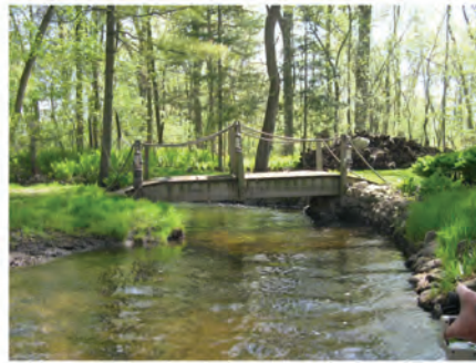
30- FOOT BRIDGE (RM 0.04 )
