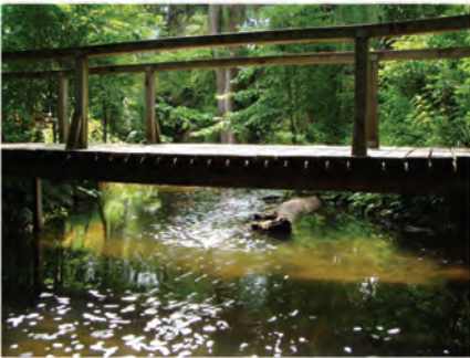
47- FOOT BRIDGE (RM 1.33)
