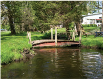
29- FOOT BRIDGE (RM 0.02)
