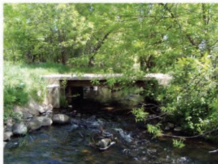
33- FOOT BRIDGE (RM 1.86)
