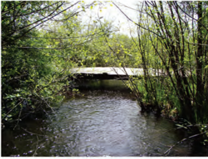
38- FOOT BRIDGE (RM 2.52)
