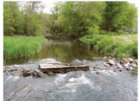
34- FOOT BRIDGE (RM 1.99)
