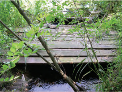
44- DAM/ACCESS ROAD (RM 5.63)
