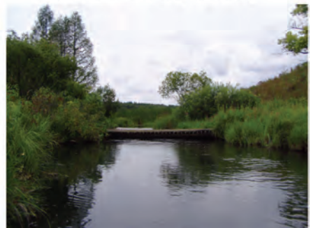
25- FOOT BRIDGE (RM 13.40)
