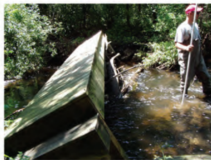
36- FOOT BRIDGE (RM 2.29)
