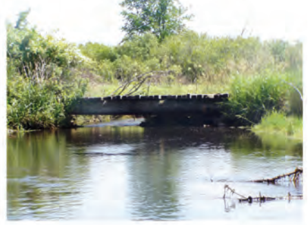
40- FOOT BRIDGE (RM 3.33)
