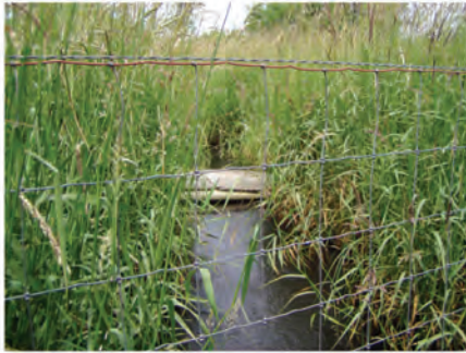
42- FOOT BRIDGE (RM 4.74)
