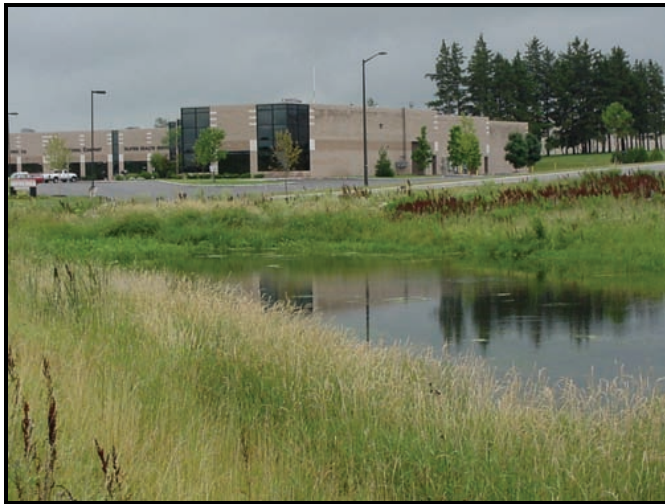
Detention basins are designed to accommodate stormwater runoff.
