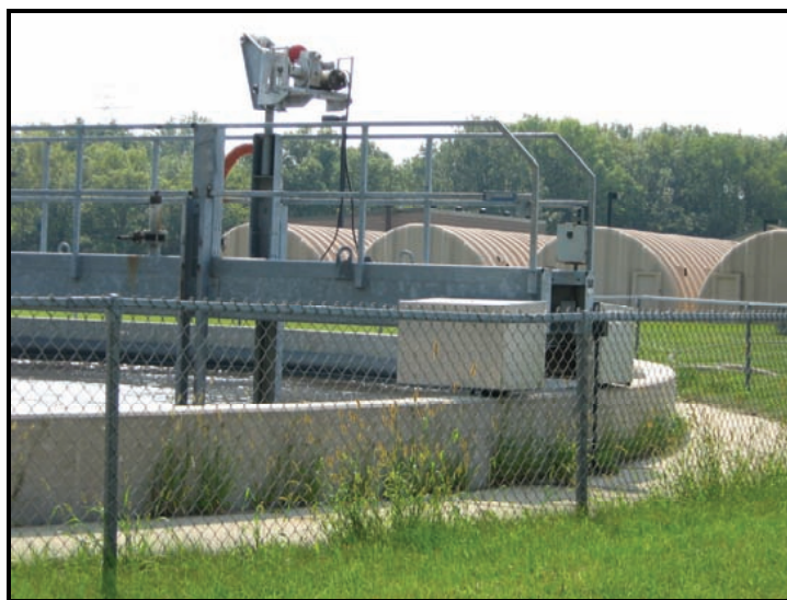
The municipal sewage treatment plant in the Village of Jackson.
