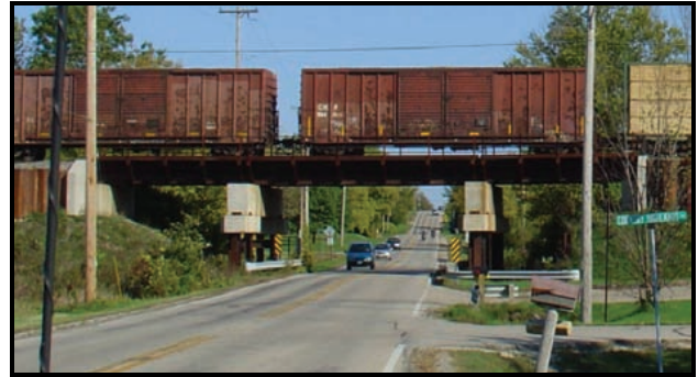
Washington County should continue the countywide bridge inspection program in cooperation with local governments.
