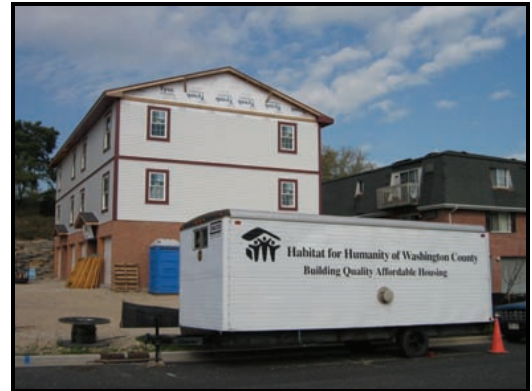
A multi-family home under construction by Habitat for Humanity.
