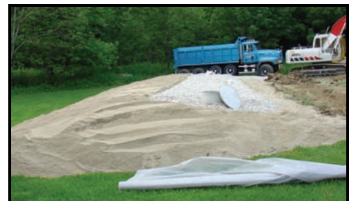
There are several different types of POWTS including at-grade, conventional systems, constructed-wetland, dripline, in-ground pressure, mound systems, and holding tank systems. A mound system is shown in the above photo.
