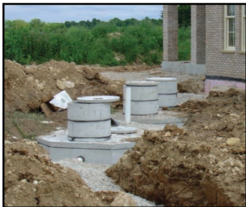
Washington County regulates private on-site wastewater treatment systems (POWTS) for any development in the County that is not served by a public sanitary sewer system.
