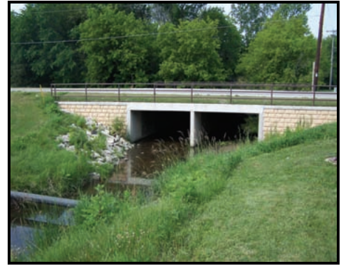
The County currently provides bridge inspection and consultation services to all local governments.
