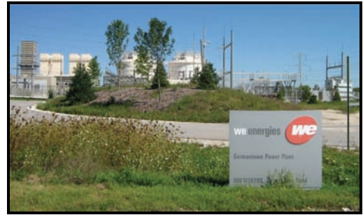
Most of Washington County is provided with electric power service by We Energies.
