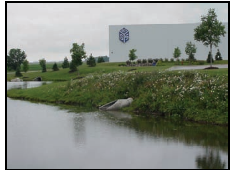
Washington County supports the implementation of water control plans, regulations, and facilities to manage stormwater runoff and flooding.
