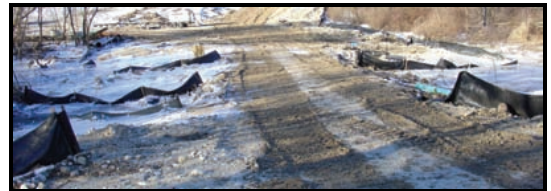
Silt fences are a method for controlling construction site pollutants.
