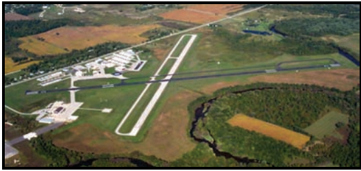
An expansion of the West Bend Airport is being considered, but is contingent upon an environmental impact study.
