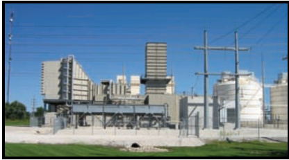
Electrical power is available throughout the County on demand and is not currently nor anticipated to be a constraint to development during the comprehensive plan design period.
