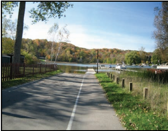
Completed boat launch facility at Henschke Hillside Lake Access on Silver Lake.
