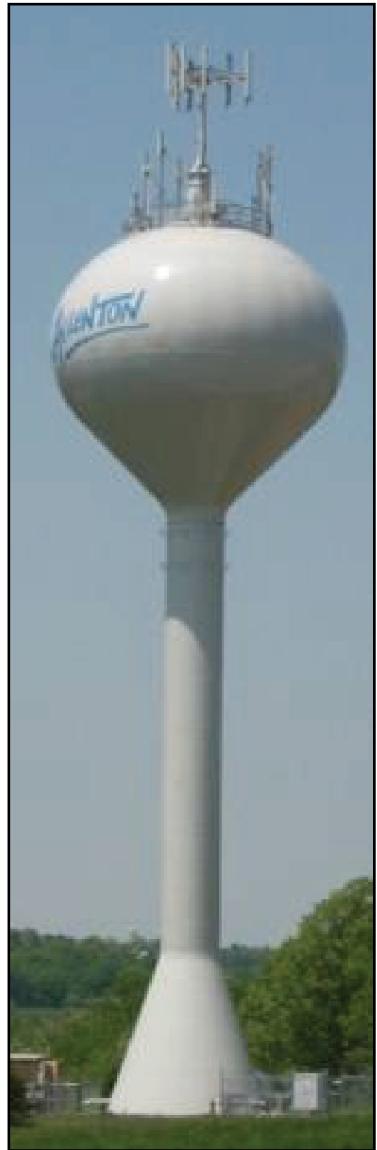
There are seven public water utilities in the County, serving 13,800 acres and 66,800 County residents in 2000. In 2004, approximately 6.7 mgd of water was pumped for use in these seven systems.
