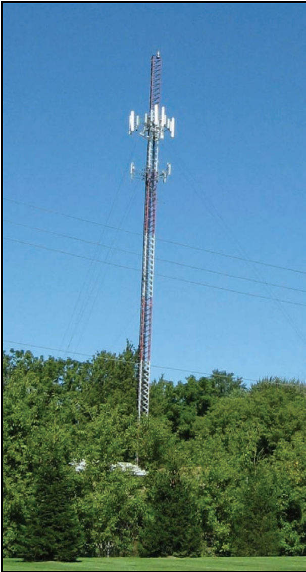
Antennas providing wireless cell phone service were inventoried in 2005 as part of the regional telecommunications plan.
