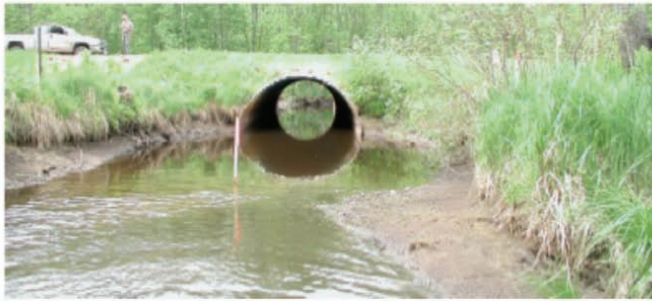
Undersized culvert
