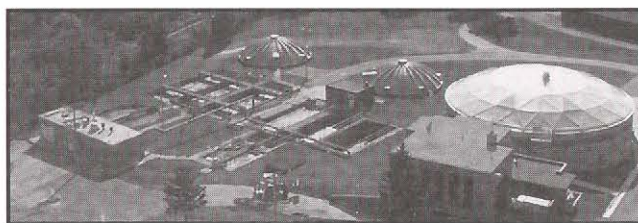
KEWASKUM SEWAGE TREATMENT PLANT
