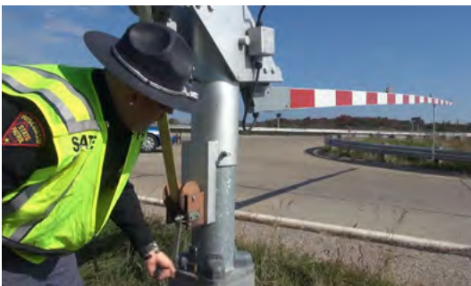
A Ramp Closure Device Credit: WisDOT
