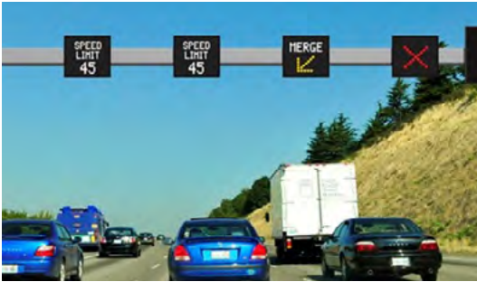
Lane Use Control Signals Credit: WSP/Parsons Brinckerhoff
