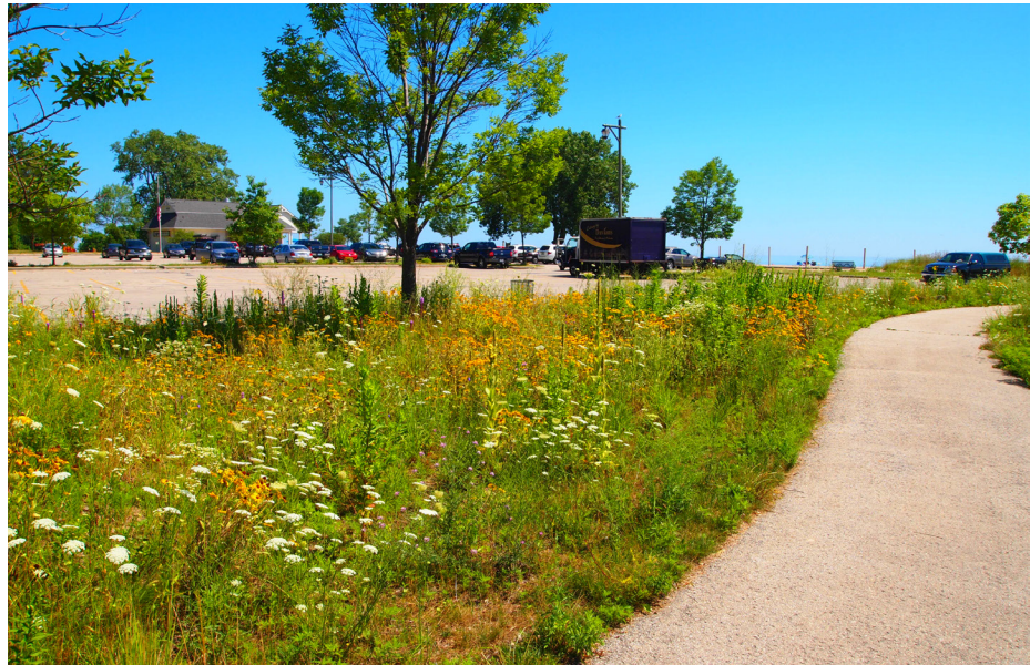
Bioswale Promoting Native Plant Species that Requires Management to Protect Against Invasive Species
