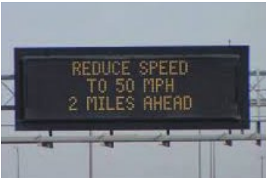
A Variable Message Sign Credit: WisDOT
