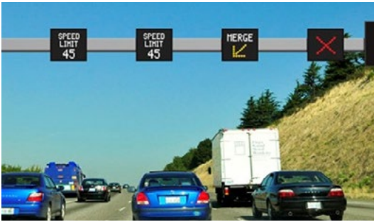
Lane Use Control Signals Credit: WSP/Parsons Brinckerhoff
