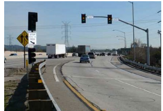
A Ramp Meter Credit: Caltrans
