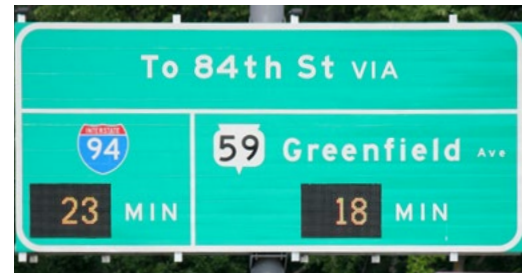
A Hybrid Variable/Static Travel Time Sign Credit: SEWRPC
