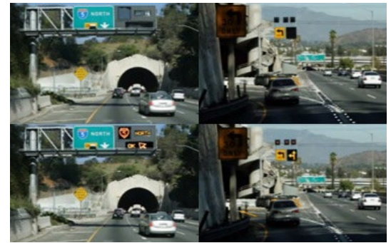
Dynamic Message Signs Show Junction Control Activated (bottom) and Not Activated (top) Credit: Caltrans
