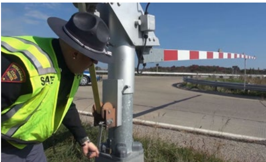
A Ramp Closure Device Credit: WisDOT
