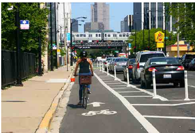
A one-way protected lane utilizing bollards to create separation for bicyclists on Kinzie Street in Chicago, Illinois Credit: Chicago Department of Transportation
