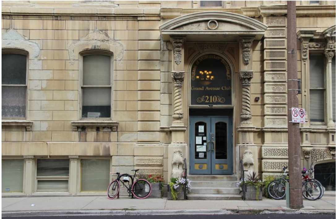
Bank of Milwaukee Building by Daniel Adams
