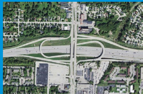
Modernization with Added Capacity
