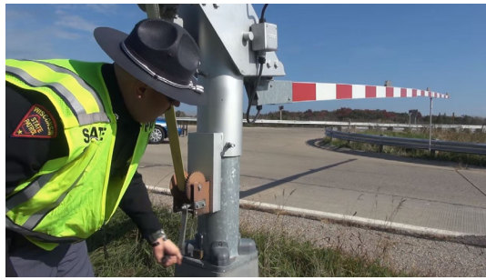
A Ramp Closure Device Source: WisDOT
