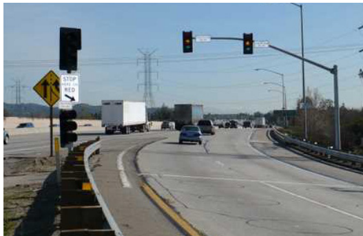
A Ramp Meter Source: Caltrans
