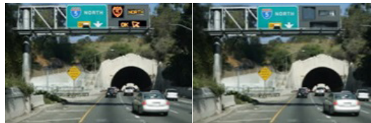
Dynamic message sign displays a junction control activated (left) and not activated (right)
