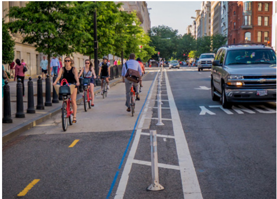
A two-way protected bike lane utilizing bollards in Washington, DC Source: People for Bikes
