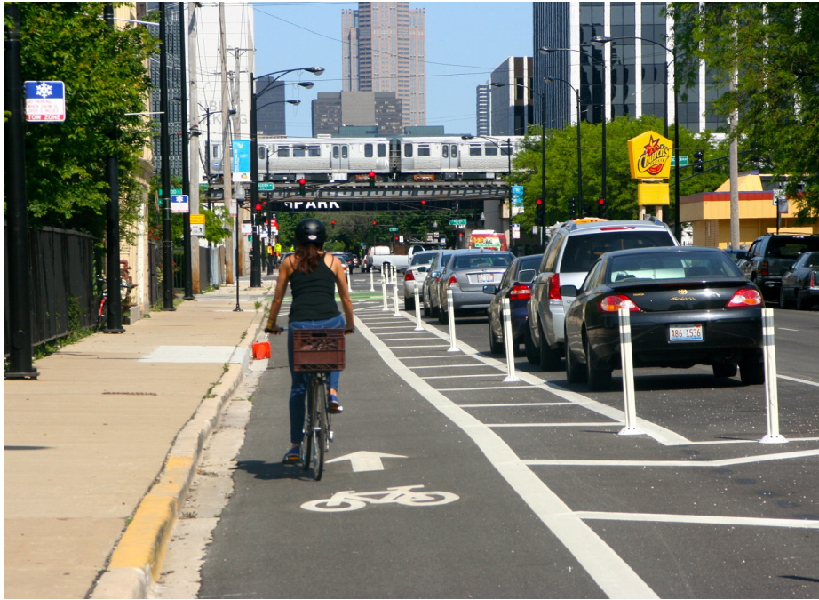
A one-way protected lane utilizing bollards to create separation for bicyclists on Kinzie St. in Chicago, IL Source: People for Bikes
