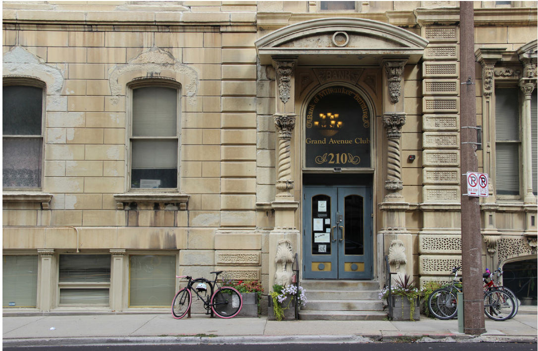
Bank of Milwaukee Building by Daniel Adams
