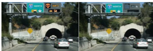
Dynamic message sign displays a junction control activated (left) and not activated (right) Source: Caltrans
