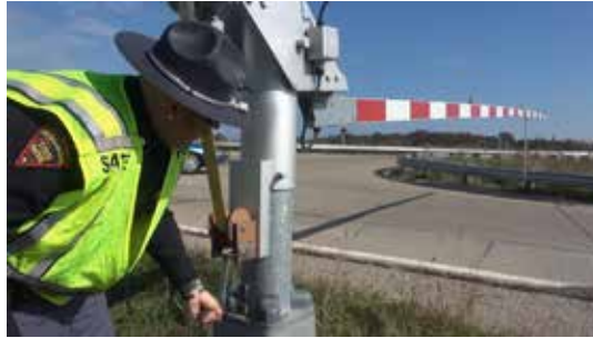
A Ramp Closure Device
